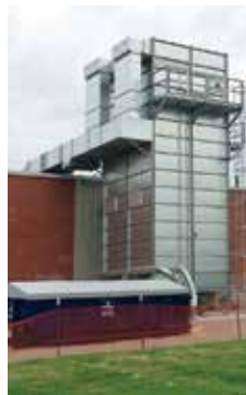
MultiStar filter installation with warm air recirculation and pneumatic transport into chip container
