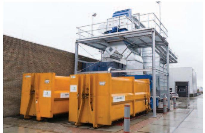
**Extraction of diecut waste via separators into stationary compactors.**
