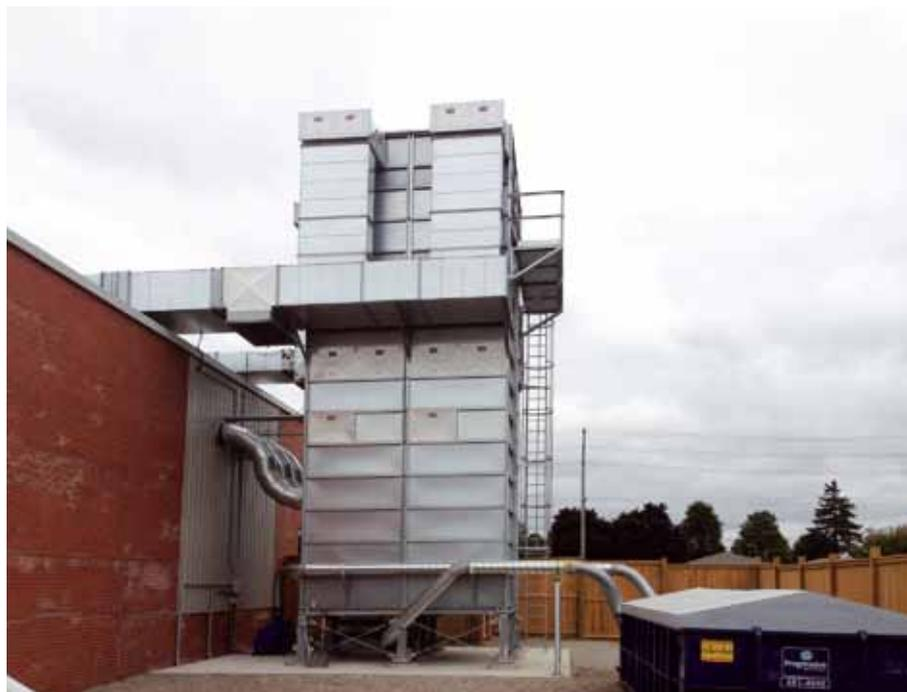
MultiStar filter installation with warm air recirculation and pneumatic transport into chip container
