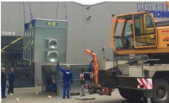
The crane in action
