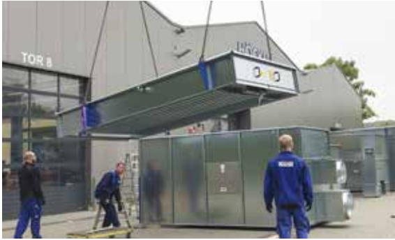
Place roof module on filter module and screw together
