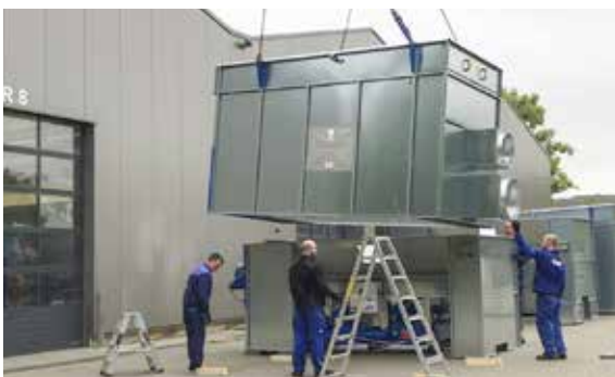
Place the two upper modules on the discharge module
